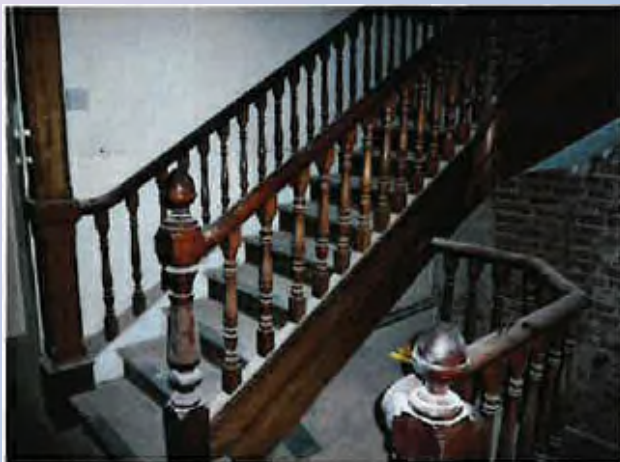
Ground Floor Rear Stair
