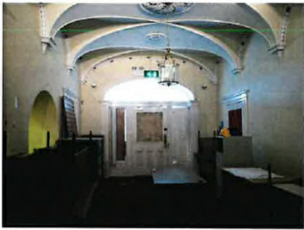
Main Hallway (Room R101)
