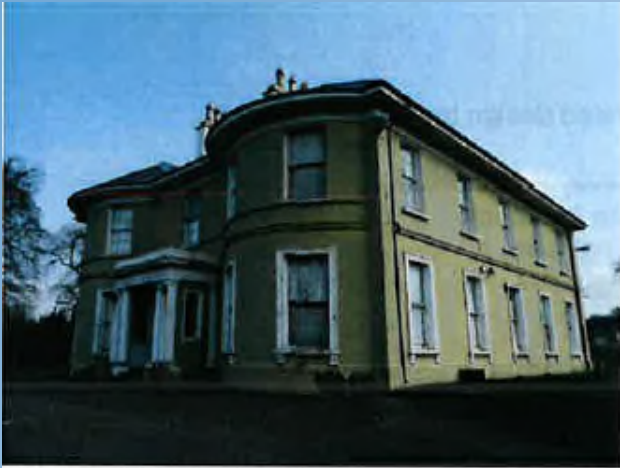
West and South Elevations
