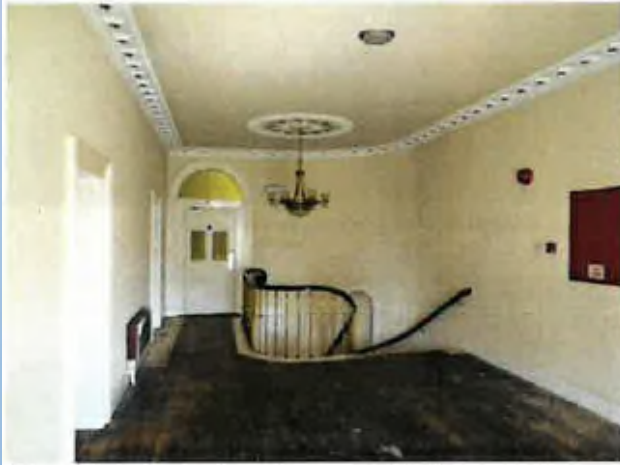
First Floor Landing (Room R201)
