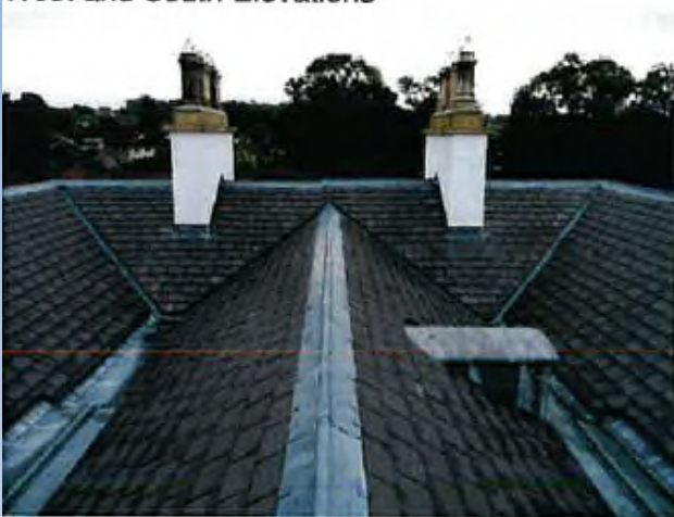
Roof (looking east)
