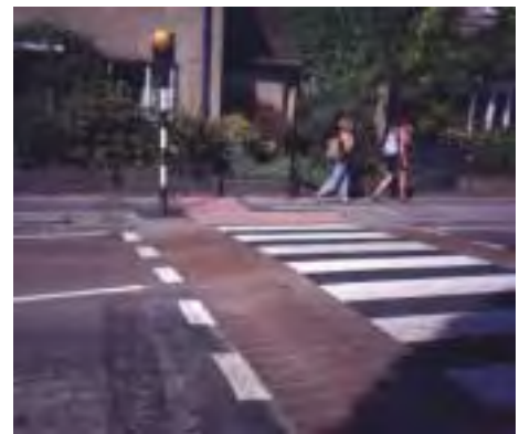
Accessible raised pedestrian crossing, also forming a flat-topped hump to slow down traffic.
