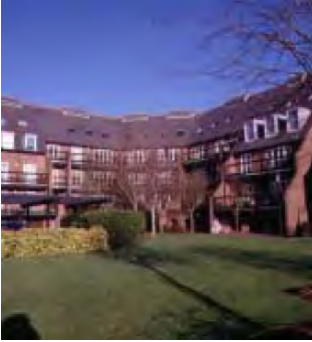
Attractive private communal gardens providing an effective contrast with the adjacent high-density apartments.
