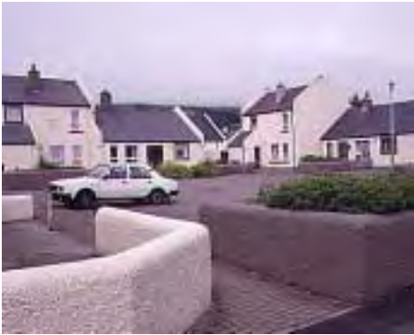
Housing in a village designed to respect rural character with the buildings enclosing and defining a shared surface space.
