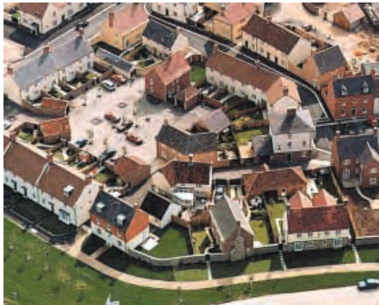
Rear access parking designed to be overlooked by some houses. The use of these parking courts means that traditional streets fronting directly onto footways can be designed.
