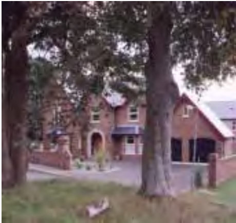
This layout was carefully designed to enable the retention of mature trees.
