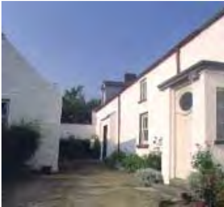
Traditional grouping of buildings.
