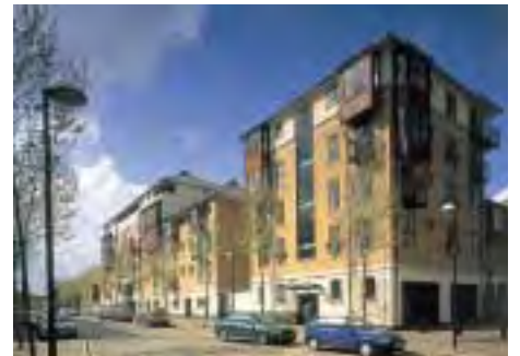
Footways on both sides of the road with trees forming an avenue.
