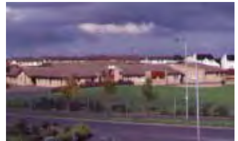
Community buildings, such as schools can act as focal points in a development.
