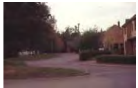
One footway omitted with single sided development fronting towards an attractive planted verge.
