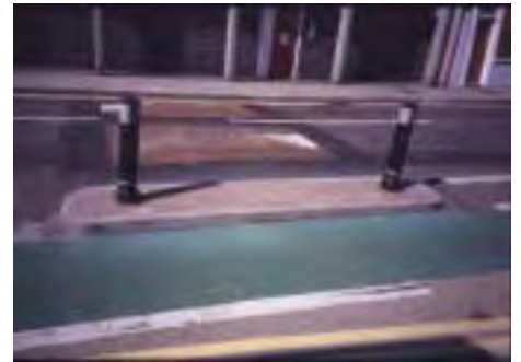
Speed cushions, pedestrian refuge and cycle lanes.
