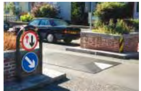
Speed cushion used in conjunction with a carriageway narrowing.
