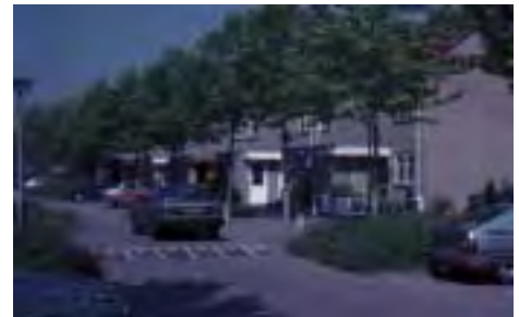
Use of a flat-topped hump as an integral part of housing design in the Netherlands.
