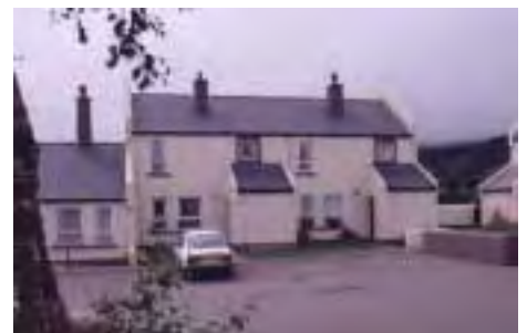
No footways - a shared surface housing square.
