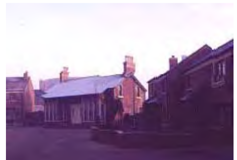
A listed building well integrated with new housing.
