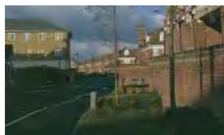
An example of a high quality rear boundary wall treatment with planting adjoining.
