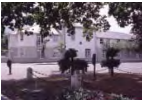
Existing building converted and extended to provide apartments.
