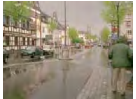
Speed restraint measures integrated with the design of a main street in Germany.
