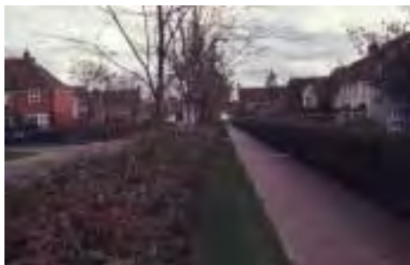
Use of verges can enhance the development and the safety of pedestrians and cyclists.
