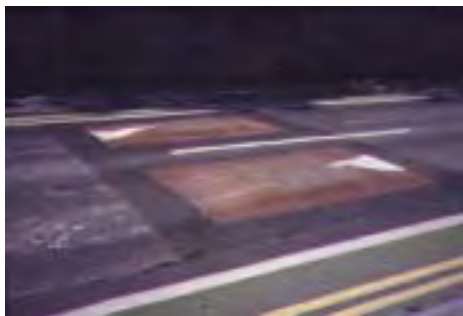
Speed cushions are the preferred method of vertical displacement on bus routes.
