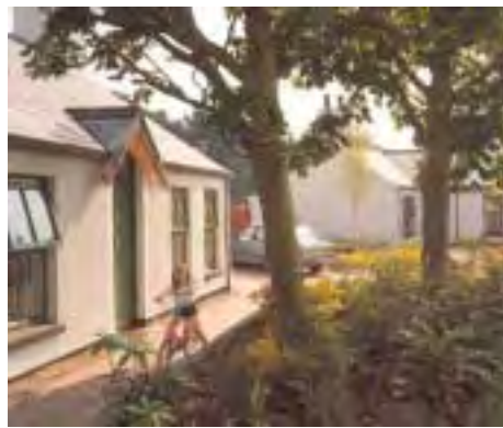
Building too close to existing trees can create significant amenity problems. These trees have now been removed.
