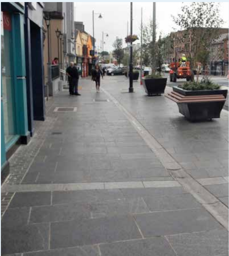
Image of high quality natural stone paving - Dark Grey Granite with Silver kerbs, trims and channels.
